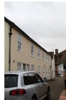
Figure 44 Narrow street at Church Square
