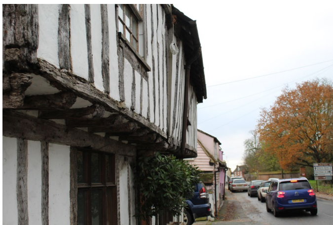
Figure 29 Street scene in Character Area 1
