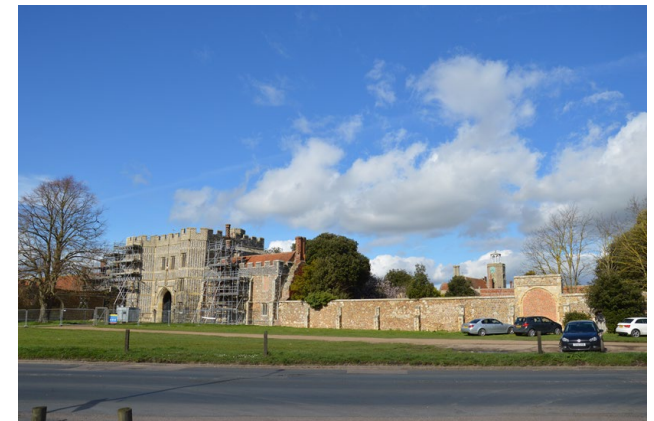
Figure 71 Flushwork of the Priory gatehouse
