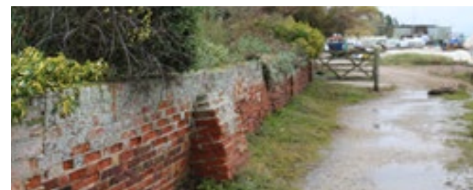
Figure 60 Example of historic walls
